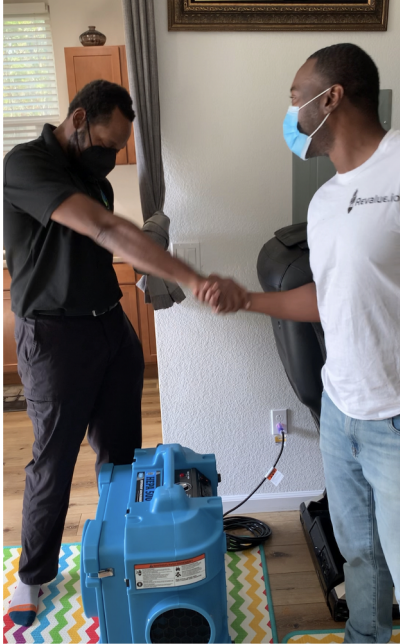
Above: East Bay Indoor Environmental works to install air filtration system
