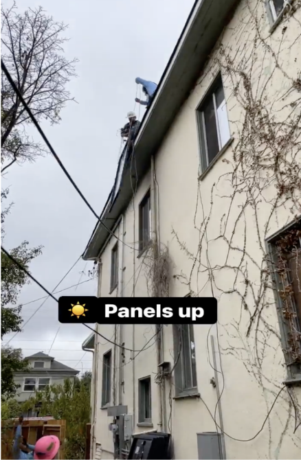
Above: Solar Panels being installed during Green Healthy Home Renovation
