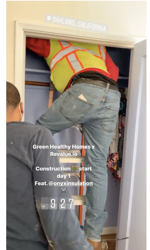
Above Right: Construction start day 1 with Onyx Insulation
